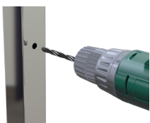
Drill hole in post to accommodate Paris offset bracket
